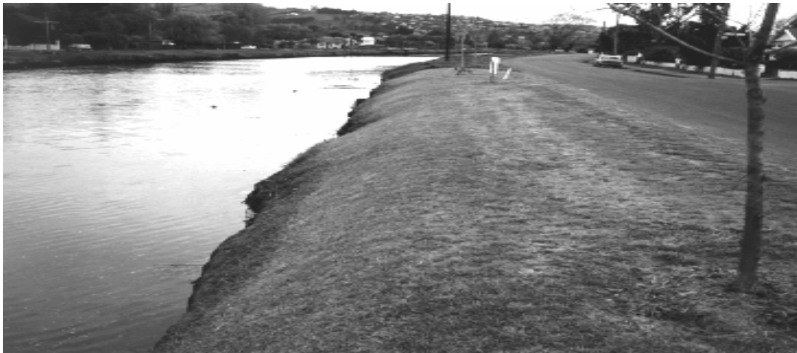
A waterway would have previously been piped or managed in a very utilitarian fashion.
